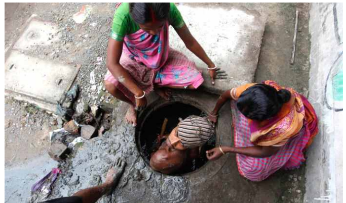
A labourer cleans an underground drain in Kolkata.
